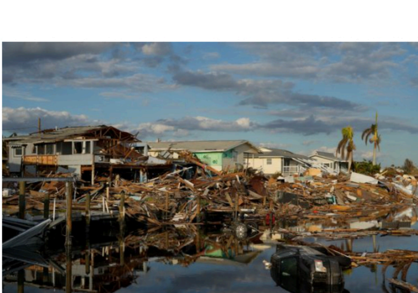
Cars and debris from washed-away homes line a canal in Fort Myers Beach, Fla., in the wake of Hurricane Ian. PHOTO: REBECCA BLACKWELL/ASSOCIATED PRESS
